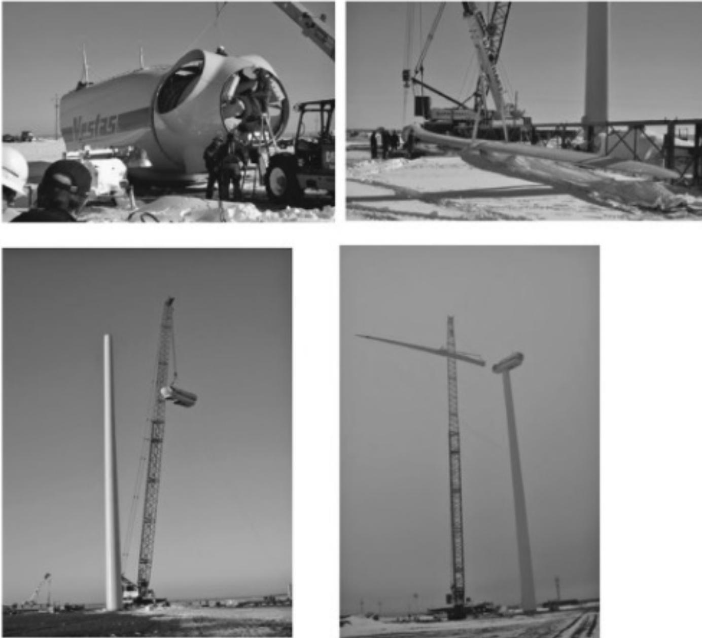
**FIGURE 6.23** Photos showing stages of erection of 3-MW wind turbine.
