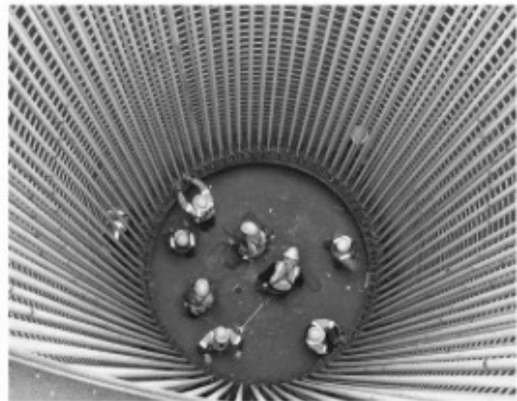
**FIGURE 6.22** Pier foundation, concentric cans, for 3-MW wind turbine. Right: bolt rods are in place and starting to attach rebar.
